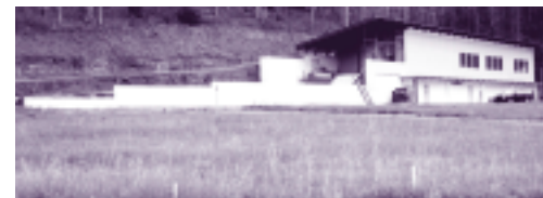
2000 First construction stage (3,600 sq. ft.) of Morrow Branch production facility completed.
