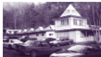
1988 7,000 sq. ft. factory & office space constructed.
