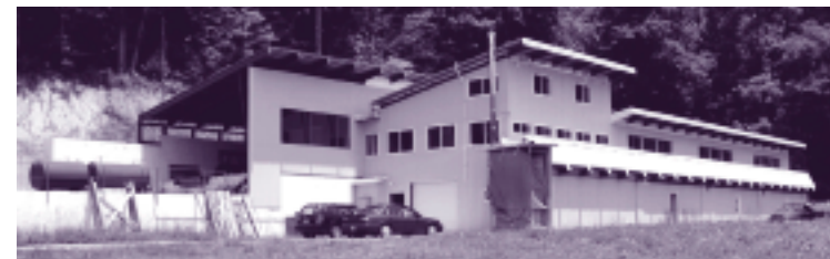
2004 Second construction stage (4,500 sq. ft.) of Morrow Branch production facility completed.
